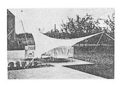
Fig 2.3 Minimum Surface Bounded by 4 Cables and 2 Masts
