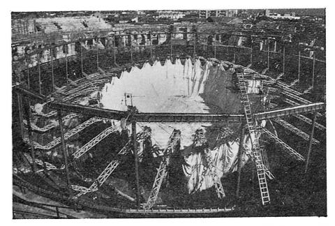
Fig. 10 Arena Nimes Membrane cushion during lifting by the help of 30 outriggers.
