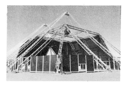
Figure 7 - Erection: installing fabric
