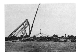
Figure 6 - Erection: raising pyramid
