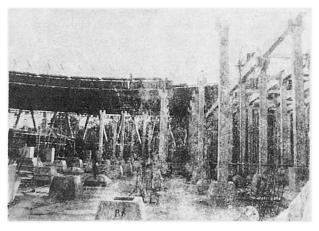
Fig. 6 Hydraulically climbing form in position.
