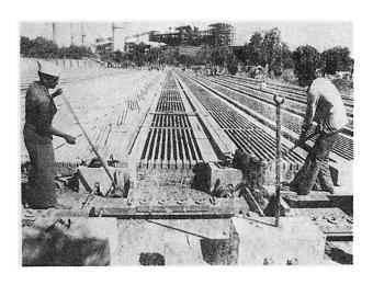
Fig.4 A typical lath-casting yard
