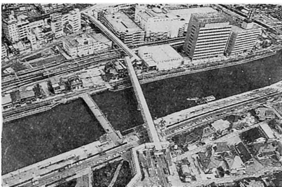
Fig.10 Modern footway promenade: Osaka
