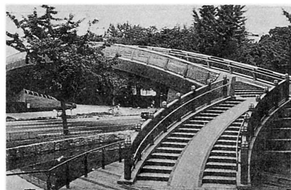
Fig.11 Modern footway bridge: Nagoya - Shirakawa
