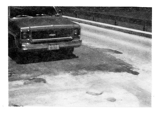
Fig.4 Bridge deck repaired by polymer concrete
