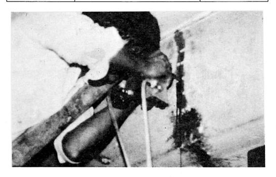
Fig.5 Building frame repaired by epoxy injection
