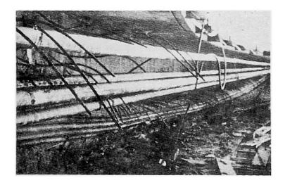
No tie-back reinforcement and inadequate cover was present to equilibrate out-of-plane forces when the tendons were stressed -- the arc became a chord. Again, minimal attention to good detailing and force paths would have prevented their collapse
