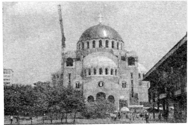
All arched shapes of the galleries and vaults have been transformed into assemblies of elements curved in two dimensions which, having been erected, form a three-dimensional shape. The semi-domes and the dome have been linearized by designing a system of arched trusses and two layers of curved decking. The precast parts are bound into a whole by in-situ cast parts of the structure which provide the required safety and long life of the building.
