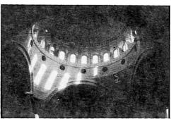
Structural connection between pendentive and main dome is to be done by supporting the dome in four position by means of hydraulic jacks capable to produce force of 3000 kN each (total force 12000 kN). These means that pendentive will take care of additional loads coming latter from applied mortar, mosaic and outside marble.
