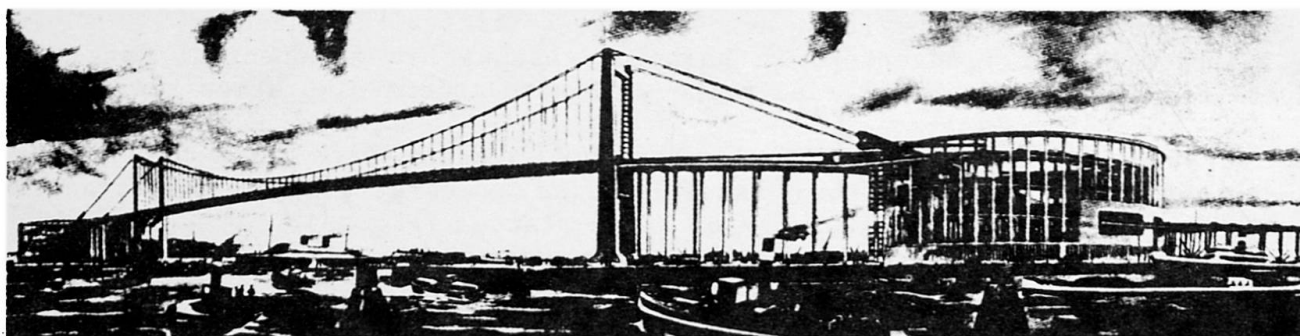
Fig.3 A bridge with spiral type access structures as proposed for the Maastunnel in Rotterdam.
