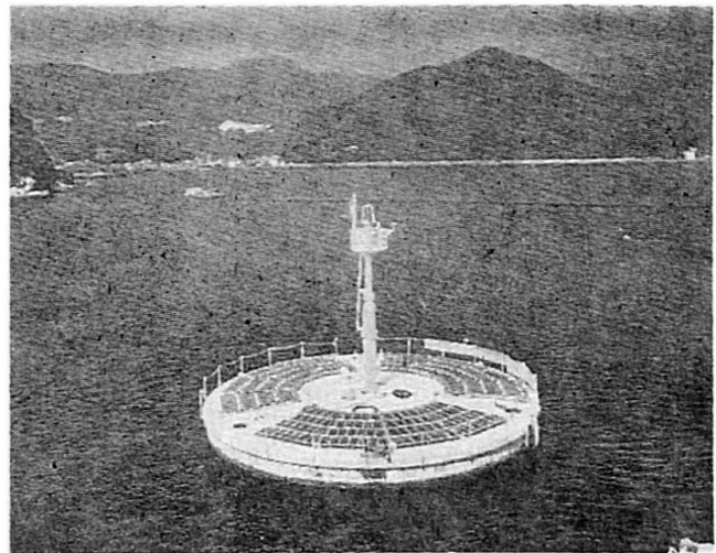
Fig. 9 Marine photovoltaic power generating system
