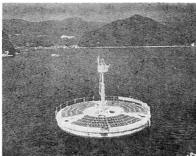
Fig. 9 Marine photovoltaic power generating system
