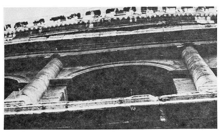
Pic.9: Sinusoidal deformations of the external wall showing the signs of the earthquake
