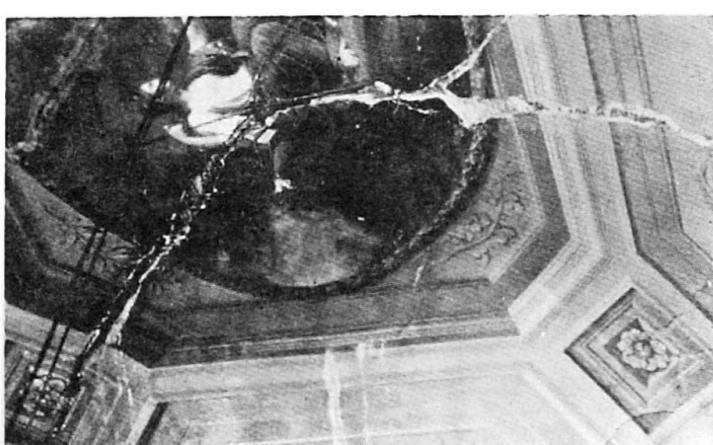
Pic.21: Cracks in the vaults of Ducal Palace of Modena
