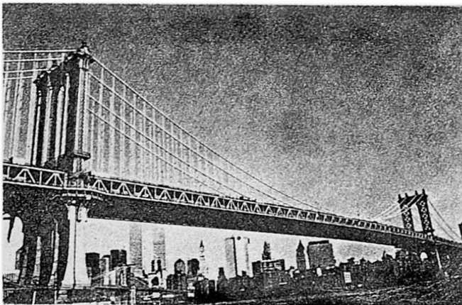
Manhattan Bridge, New York, USA
