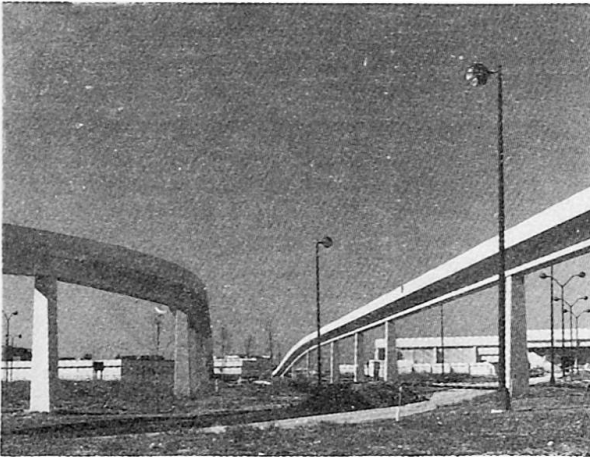
Fig 6. Straight stems and curved decks offer economy during construction at the Dallas/Fort Worth Airport.
