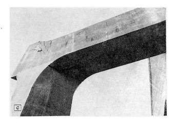
FIG 5. Earthquake Damage, Loma Prieta 89, China Basin Viaduct
