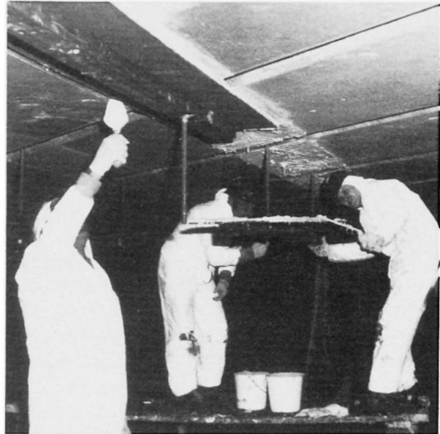
Fig. 3 Bonding of Steel Plates
