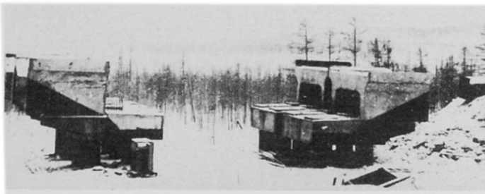
Fig. 4. Completely precast columnar pier
