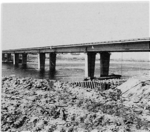
Fig.22. Continuous composite superstructure
