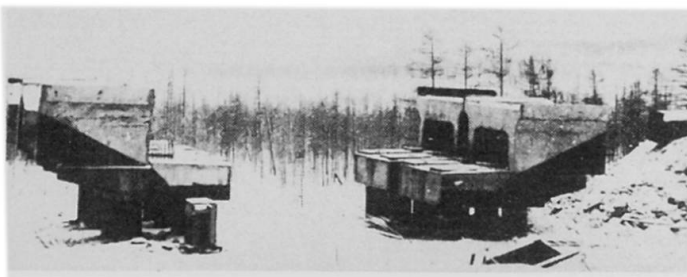
Fig. 4. Completely precast columnar pier
