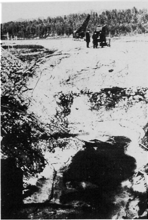
Fig. 1. Construction of foundation pit for massive pier
