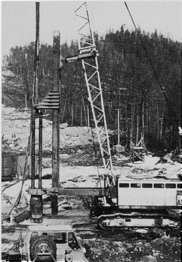
Fig. 6. Holes boring by rotary drill
