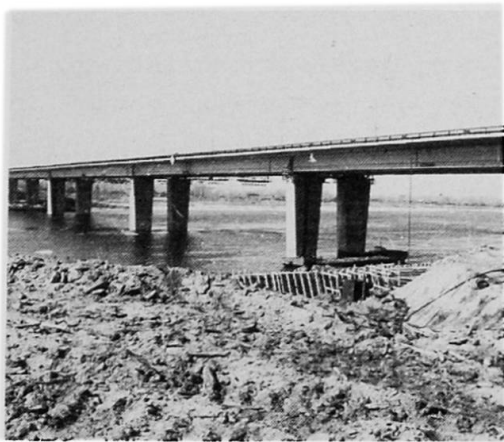
Fig.22. Continuous composite superstructure
