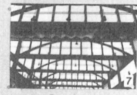
4 Lifting 40 T precast prestressed tied arch girder 30 M span. 5 Tied-arch girders erected and in position 6 6 cm thick folded plate element 12 m. 7 Folded plate elements in position
