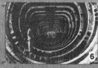
4 Shuttering for Voussoirs Voussoir partially prestressed to release trolley
