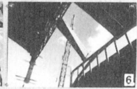
4 Lifting 40 T precast prestressed tied arch girder 30 M span. 5 Tied-arch girders erected and in position 6 6 cm thick folded plate element 12 m. 7 Folded plate elements in position
