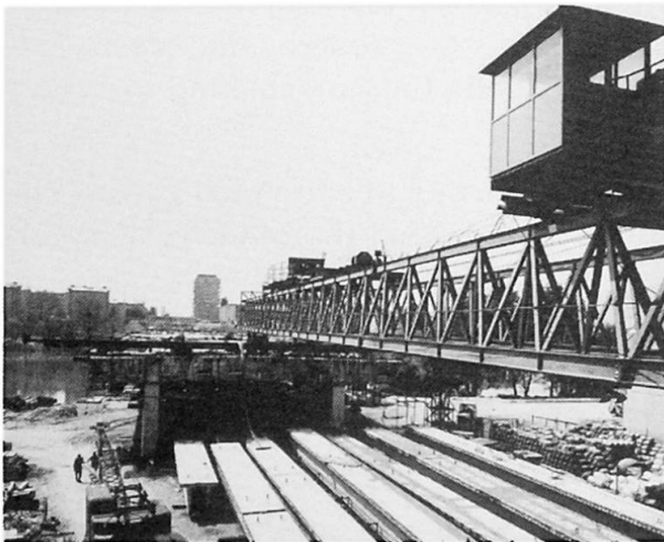
Fig. 11: Beams during grouting at the construction site.
