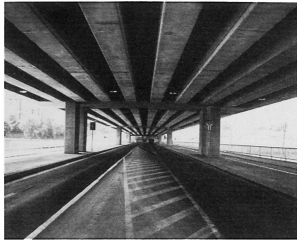
Fig. 2: The slab of the upper bridge
