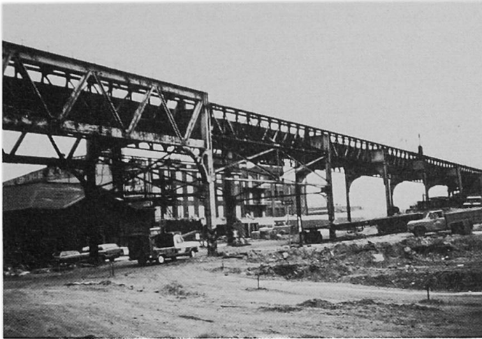
Figure 1 The built-up steel members of the Philadelphia transit system are indicative of early transit development. (Photo by author)
