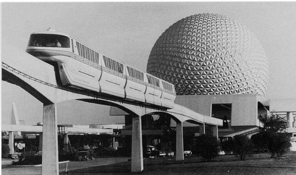
Figure 8 The Walt Disney World Monorail uses precast concrete beams and a flexible steel plate to connect the beams to the columns. The resulting structure is virtually maintenance free and close to an optimum structural design. (Photo c. Walt Disney Productions, used with permission)
