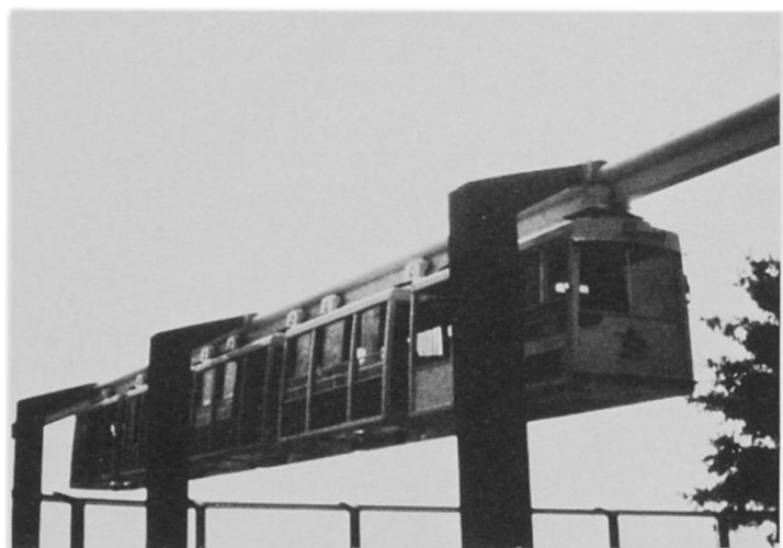
Figure 6 Busch Gardens in Tampa, Florida, uses an I-beam guideway to support a suspended vehicle. Low operating speeds allow use of a very small guideway section. (Photo by Dr. Robert Stevens, used with permission)
