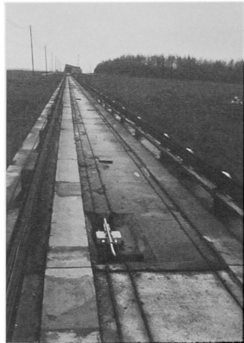
Figure 5 The Matra-Val Transit System in Lille, France, uses a precast concrete running pad for its at-grade and elevated guideway. The running pads can be equipped with heating cables for operation in ice and snow environments. Steel I-beams at the side of the guideway provide a steering surface and serve as power distribution rails. (Photo by author)
