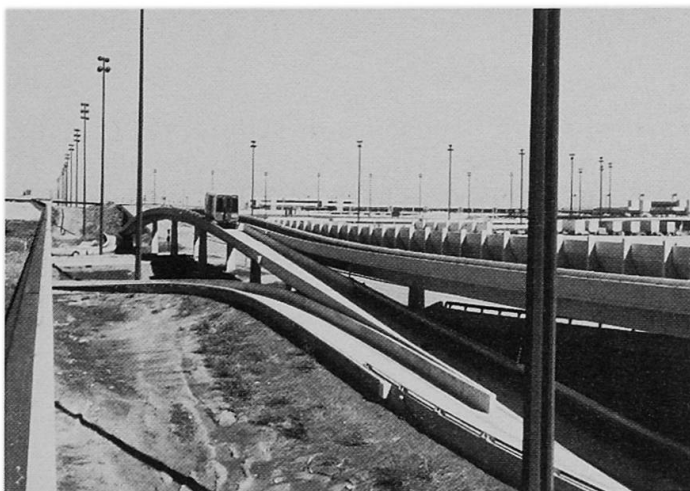
Figure 3 The Dallas-Fort Worth Airport uses a precast concrete box girder with side walls to support the transit vehicle. The vehicle steers off the top of the concrete wall. (Photo by author)
