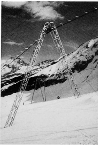
Fig. 5 Intermediate pylon
