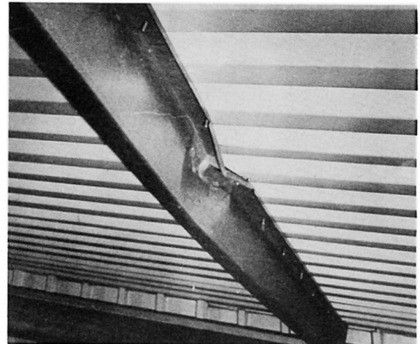
Fig.3 Buckled Z-purlin.
