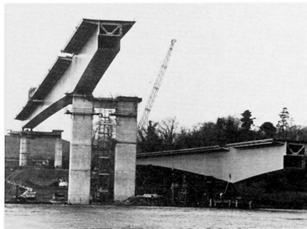
Fig. 9. Sidespan in final position
