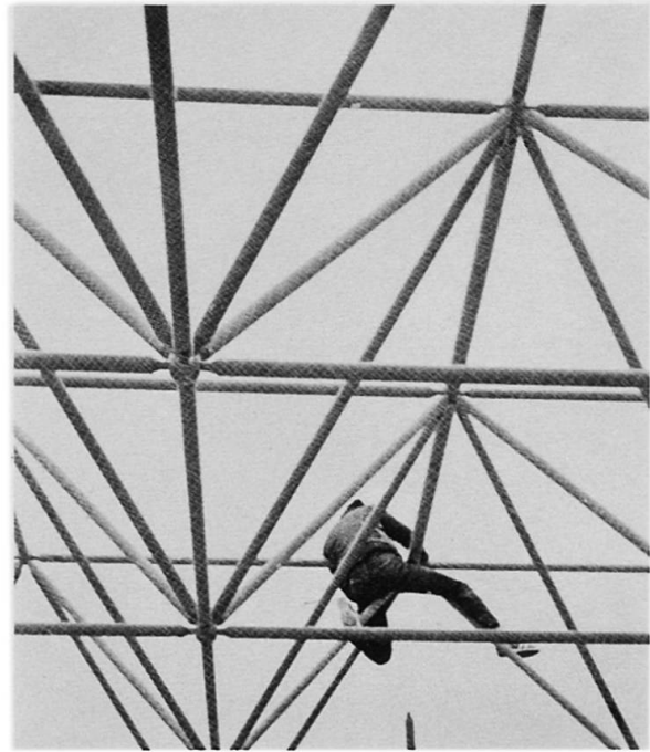
Fig. 14 Space truss of the Mero system
