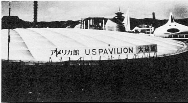
Fig. 2 U.S.A. Pavillion air supported roof at Osaka Expo 70
