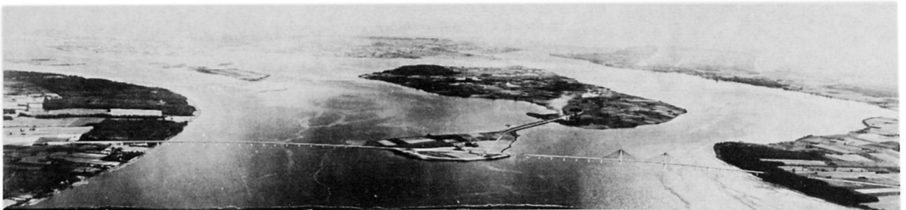
Fig. 6 Aerial view of tender project.
