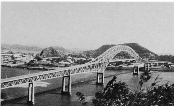
12. Thatcher Ferry Bridge over Panama Canal
