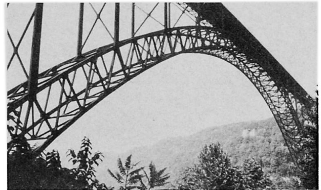
21. New River Gorge Bridge
