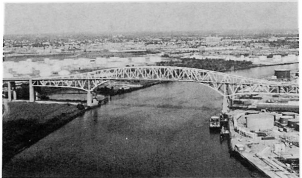
11. George Platt Bridge
