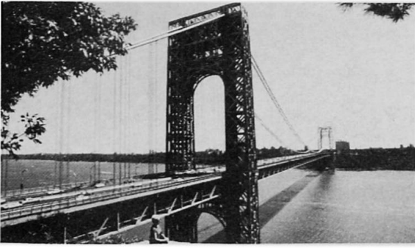
5. George Washington Bridge
