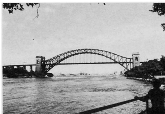
4. Hell Gate Bridge
