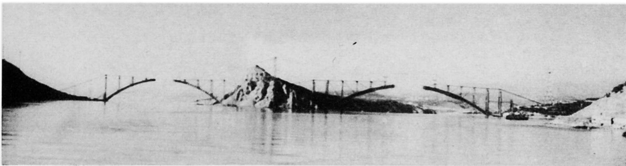
Fig. 7 - Erection of the central portion of the bridge arches
