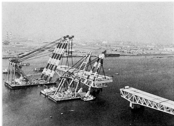
Fig. 3 Erection of the largest block (4,250 ton)
