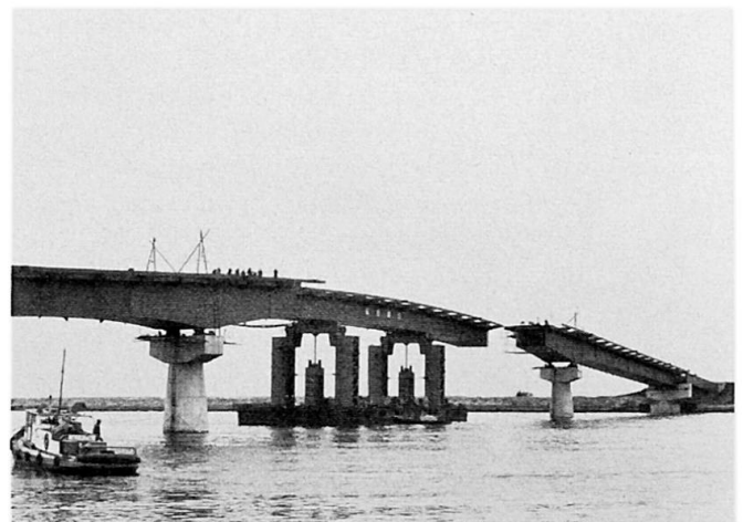
Fig. 2 Erection of a block of 605 ton by lift-up barge
