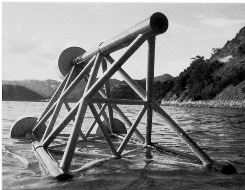
Fig 3. TRICON IS FABRICATED & FLOATED HORIZONTALLY
