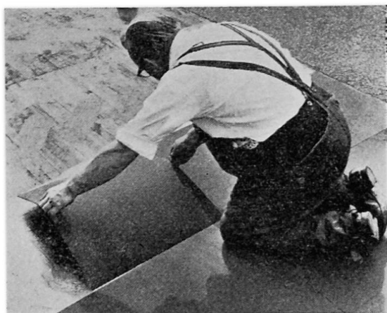
Fig. 5. Laying thin sheeting based on poly-vinyl chloride.
