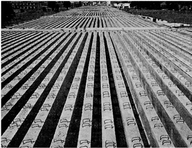
Fig. 7. Prestressed bridge beams in the Chiswick-Langley motorway.
