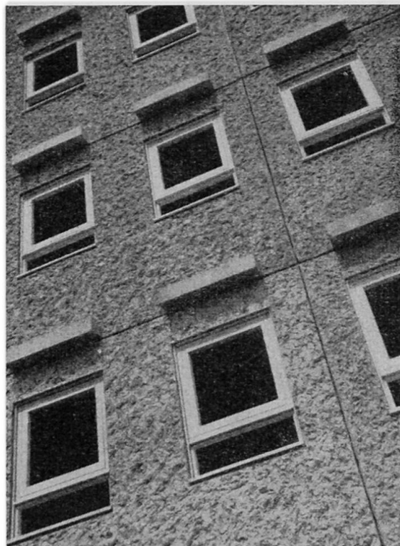
Fig. 1 - 20-storey block of flats at Smethwick of precast load-bearing walls with simulated rock finish.
