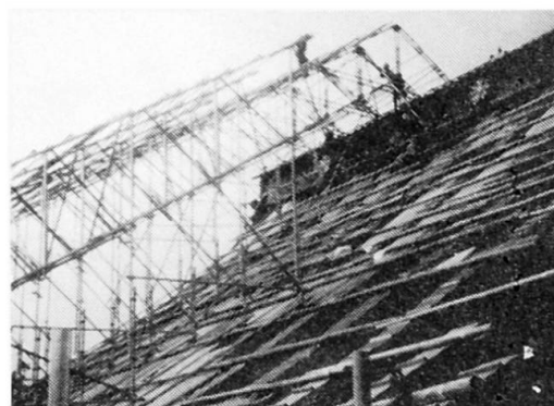
Fig.11, Kimpusanji temple, Zaodo Manual removal of roof
