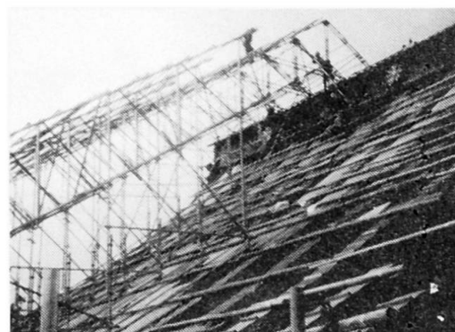
Fig.11, Kimpusanji temple, Zaodo Manual removal of roof
