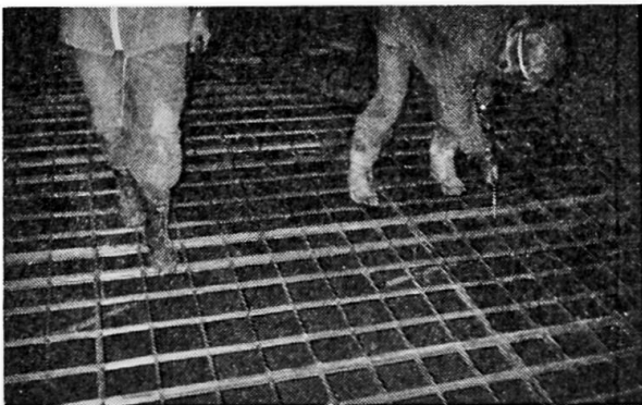
Fig. 5 Reinforcements for invert of concrete lining
