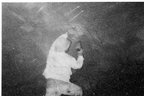
Fig. 2 Setting method of reinforcing grids for shotcrete
