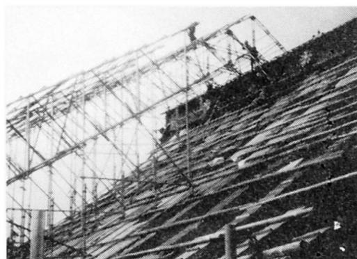
Fig.11, Kimpusanji temple, Zaodo Manual removal of roof
