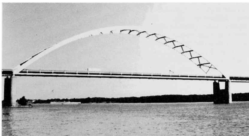
Figure 1 - View of 223 m tied-arch span.
