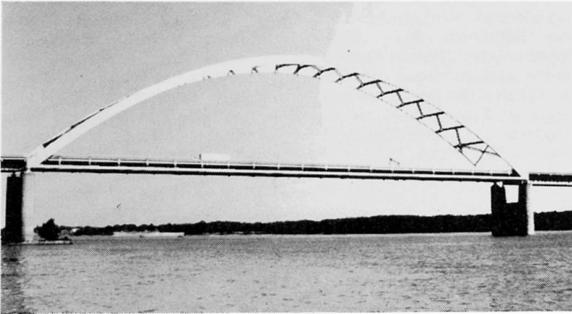
Figure 1 - View of 223 m tied-arch span.
