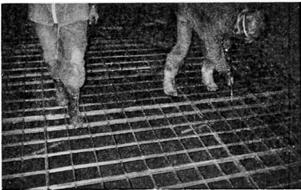
Fig. 5 Reinforcements for invert of concrete lining
