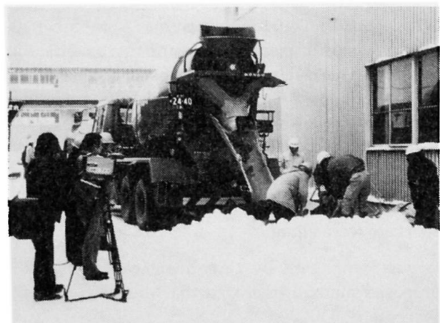
Fig. 4 Concrete placing under -5^{\circ}\text{C}
