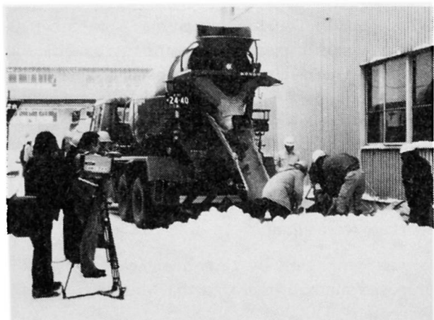
Fig. 4 Concrete placing under -5^{\circ}\text{C}
