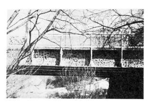
Fig.l The world's first GRP highway bridge in Ginzi, Bulgaria
