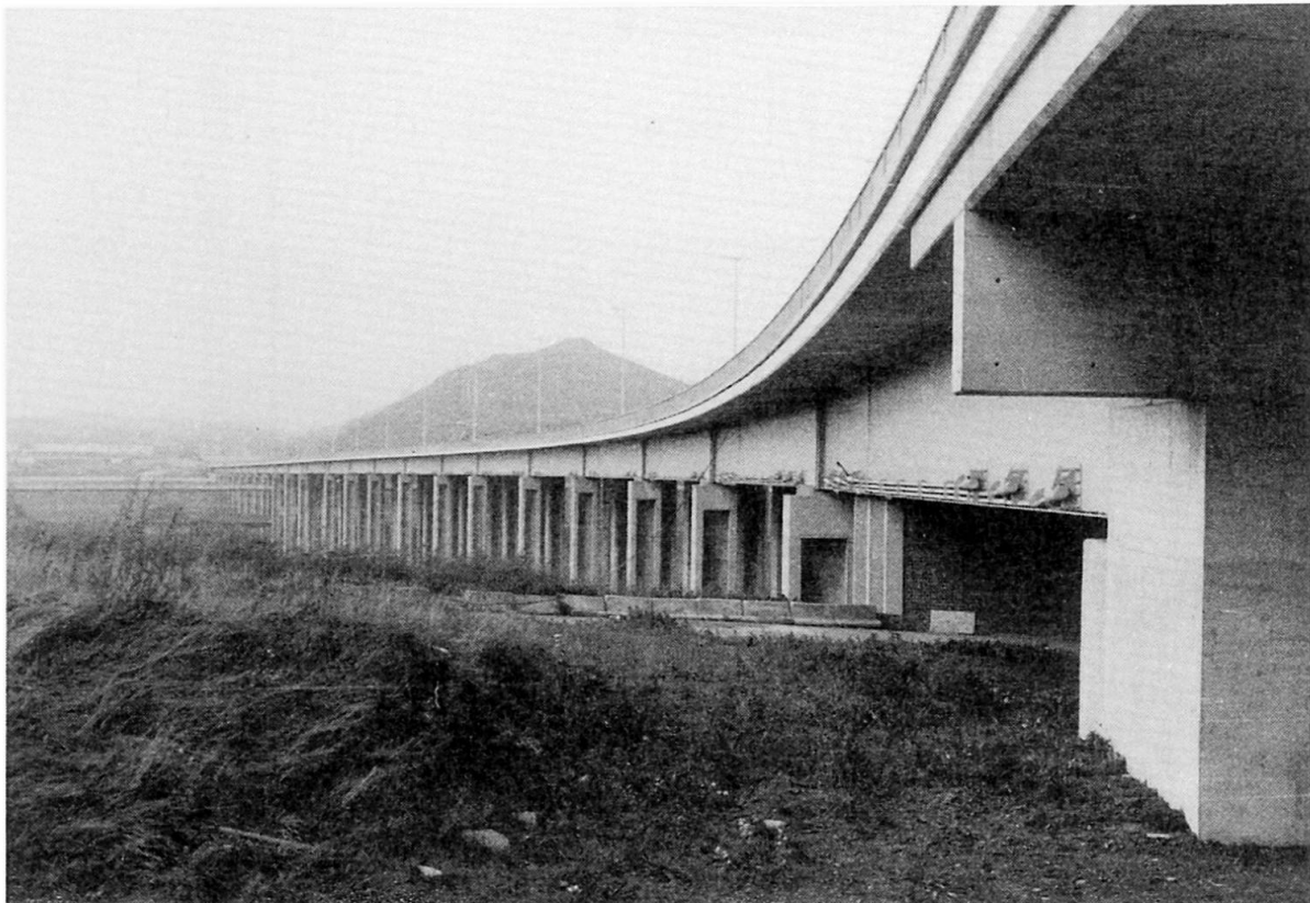
Fig 1 VIADUCT OVER THE RIVER SAMBRE AT CHATELET
