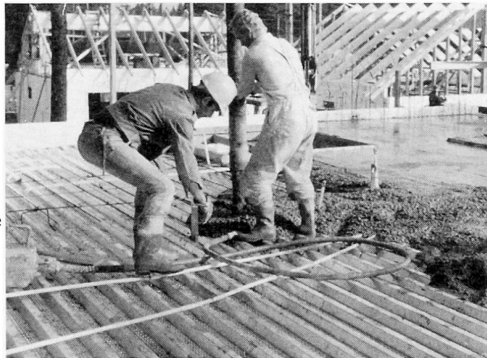
Fig.2 The fluted and spiked steel sheet is lightweight building element
