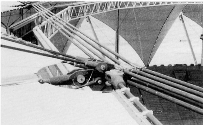
Fig. 4: Center ring detail
