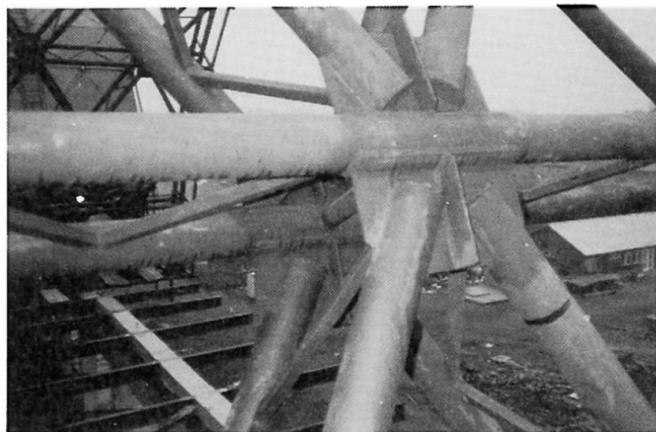
Fig. 3 Special tube-on-tube joint
