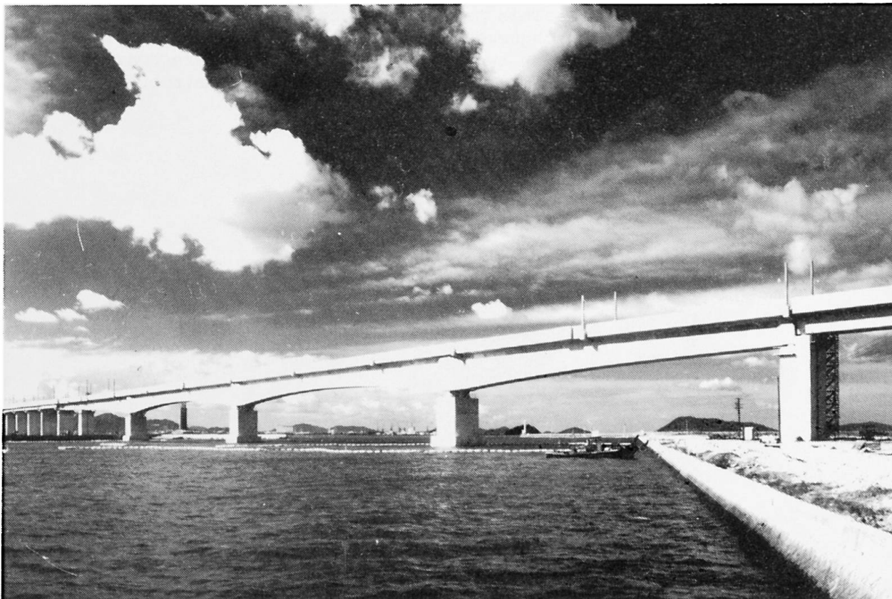
Photo-1 The completed Kitaura-ko Bridge.
