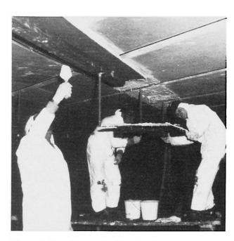
Fig. 3 Bonding of Steel Plates
