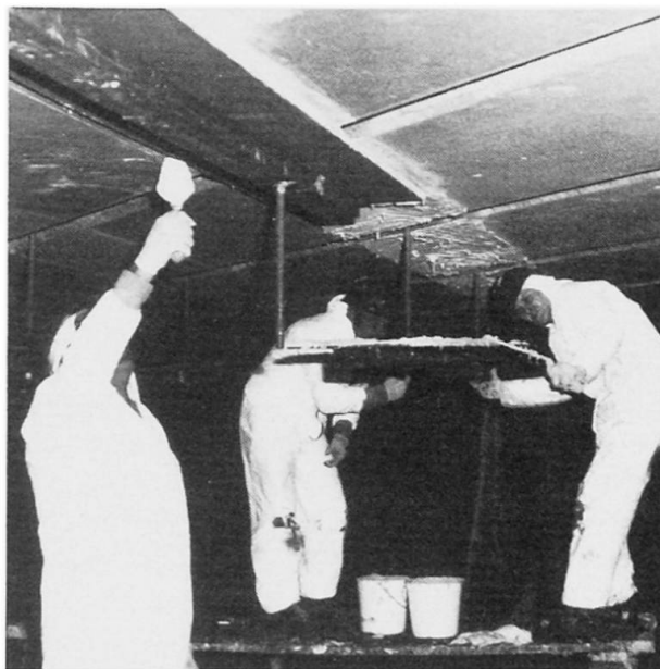
Fig. 3 Bonding of Steel Plates
