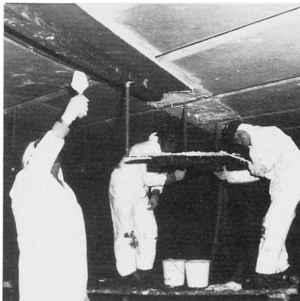
Fig. 3 Bonding of Steel Plates
