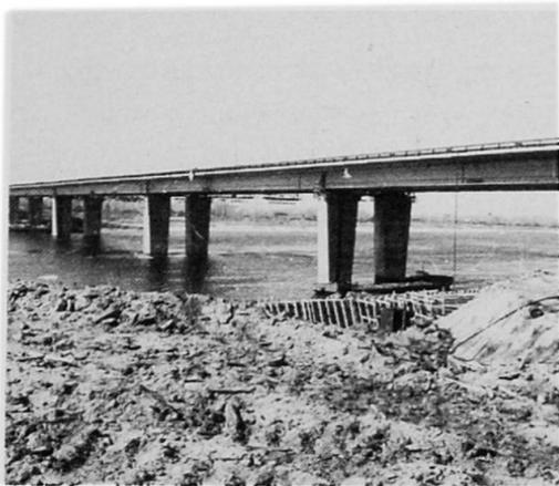
Fig.22. Continuous composite superstructure
