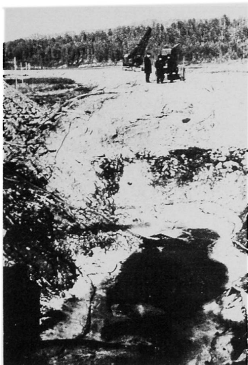
Fig. 1. Construction of foundation pit for massive pier
