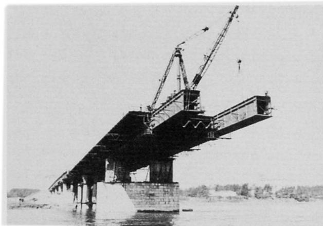
Fig.20. Continuous box girder superstructure with orthotropic deck slab
