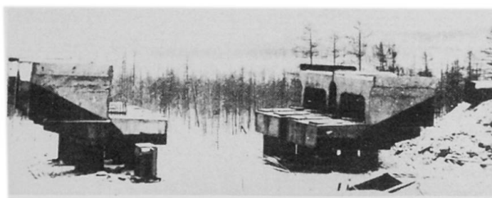
Fig. 4. Completely precast columnar pier
