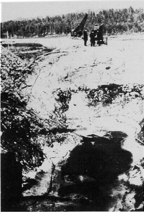
Fig. 1. Construction of foundation pit for massive pier
