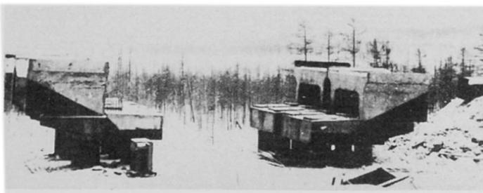
Fig. 4. Completely precast columnar pier
