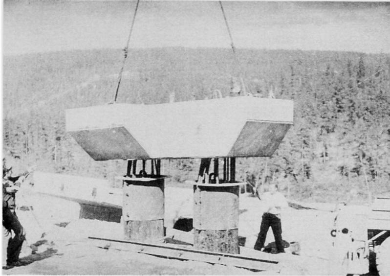
Fig. 8. Columns and caps casting
