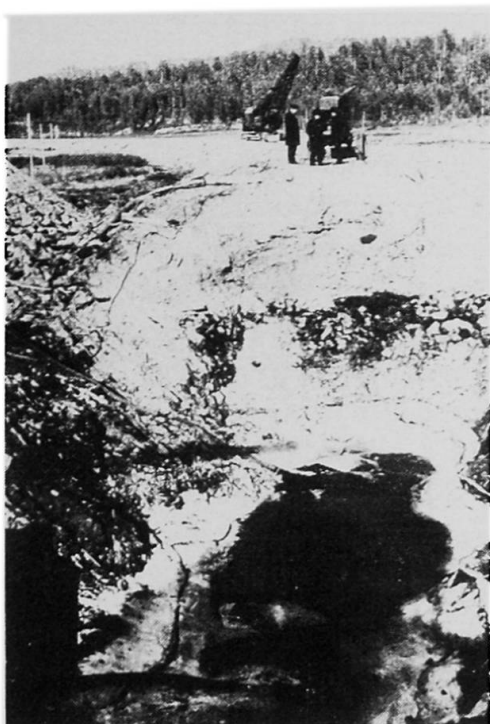
Fig. 1. Construction of foundation pit for massive pier
