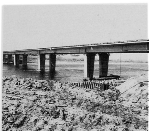
Fig.22. Continuous composite superstructure
