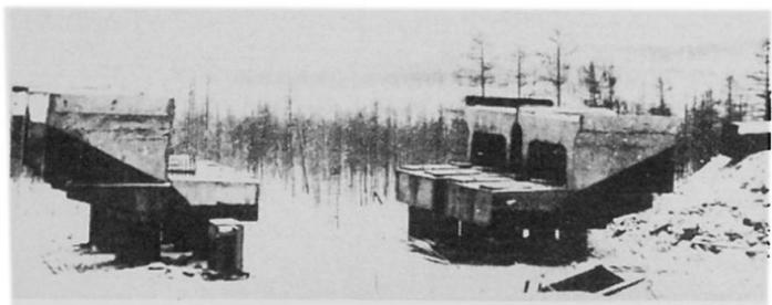
Fig. 4. Completely precast columnar pier
