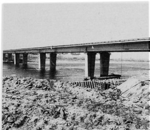
Fig.22. Continuous composite superstructure
