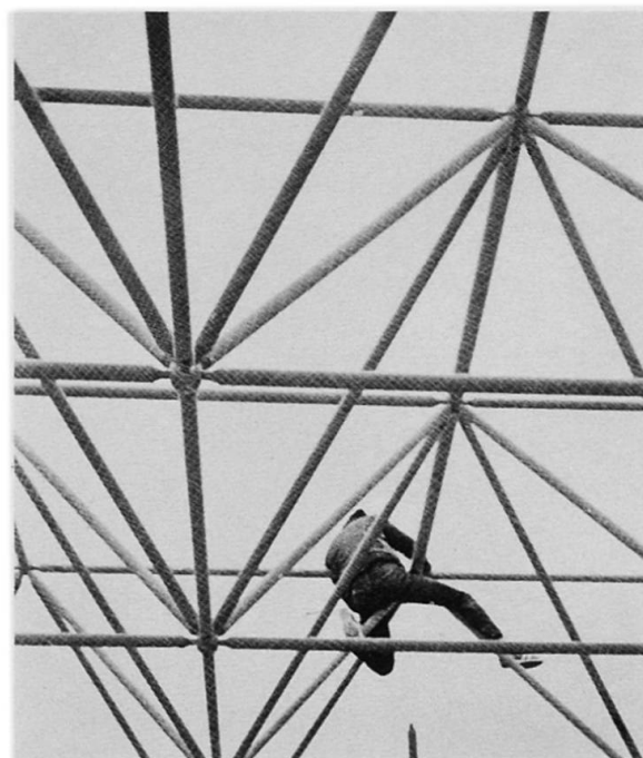
Fig. 14 Space truss of the Mero system
