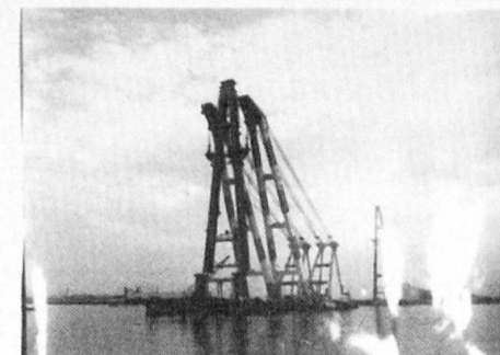
A-frame towers, the height of 104 m and the weight of 1250 ton, were hoisted into place by a 3000-ton floating crane in July, 1983.
