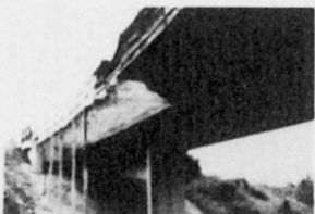
Deteriorated concrete has been removed
