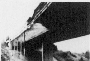
Deteriorated concrete has been removed
