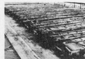
Re-established transverse prestressing.
