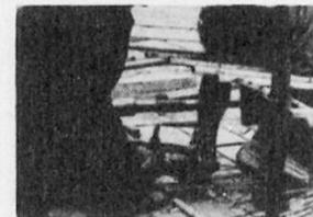
After cut-off, the 12 x 5 mm bars were prepared for coupling with simple bar anchorages. The 5 mm bars were provided with button heads on site.
