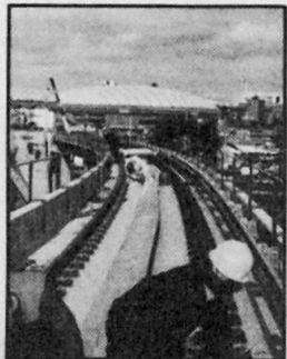
Accuracy In Beam Fabrication Permits Meeting Tight System Tolerances
