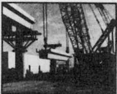
Beams Erected At The Rate Of Six Per Day
