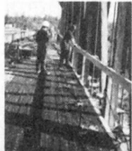
SIoux NARROWS(1982) Deck Replacement
