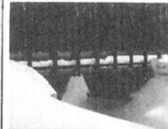
FOX LAKE Bridge New prestressed laminated wood rigid frame. Built 1981, Sudbury, Ontario.
