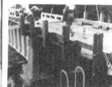
VICTORIA ISLAND Bridge. Deck replacement with prestressed wood panels. Ontario Hydro Ottawa, 1984.
