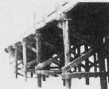
NAIL CONNECTED LONGITUDINALLY LAMINATED DECK
