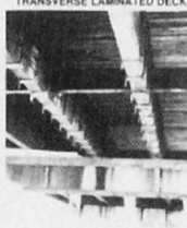
BRIDGE WITH TRANSVERSE DECKING
