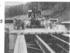
VICTORIA ISLAND Bridge. Deck replacement with prestressed wood panels. Ontario Hydro Ottawa, 1984.
