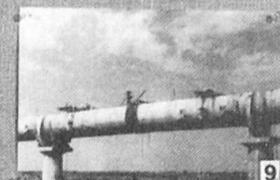
9 Key Joint concreted in situ. Prestressing of continuity cables.
