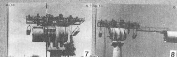
7 Cantilever lifting equipment cradles and walkway
