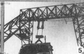
5 Specially designed equipment for handling voussoirs
